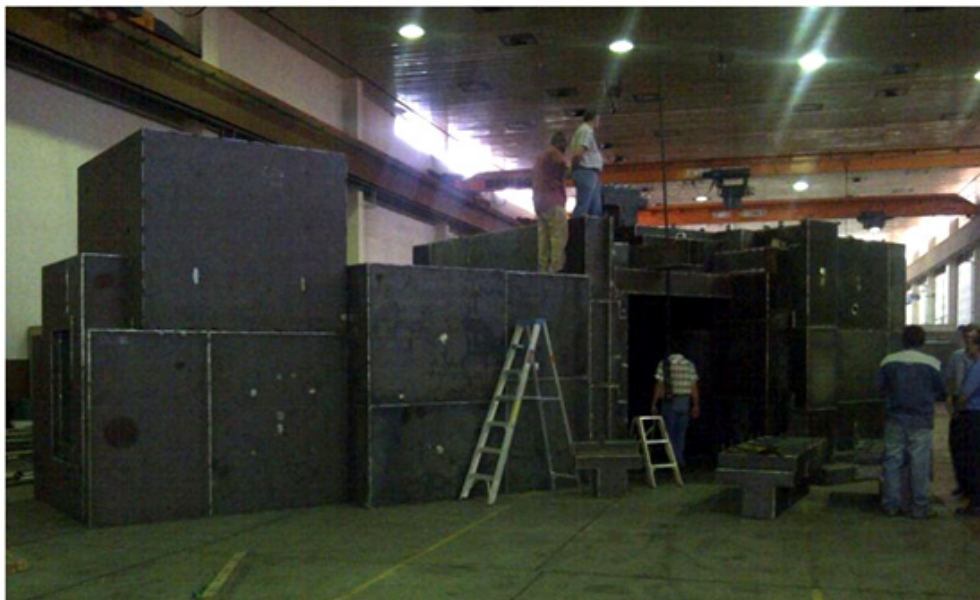
Figure 5 Mock-up facility at the manufacturing workshop at Necsa
