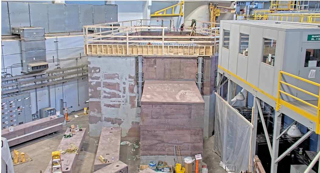
Fig. 1 VENUS instrument cave and beam stop. The roof beams are visible on the floor (left of the beam stop). Credit: ORNL, U.S. Dept. of Energy.
