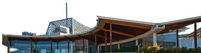
ANSTO's OPAL reactor building.
