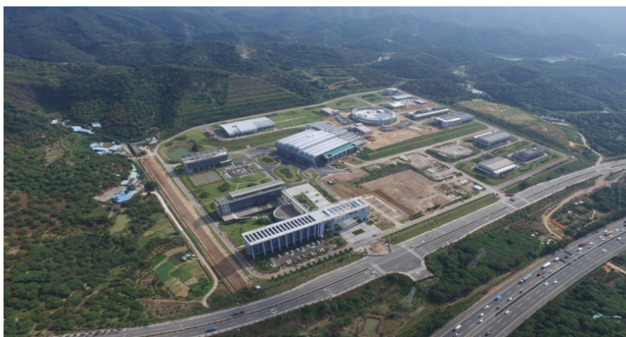
Aerial photo of the China Spallation Neutron Source taken in 2016
